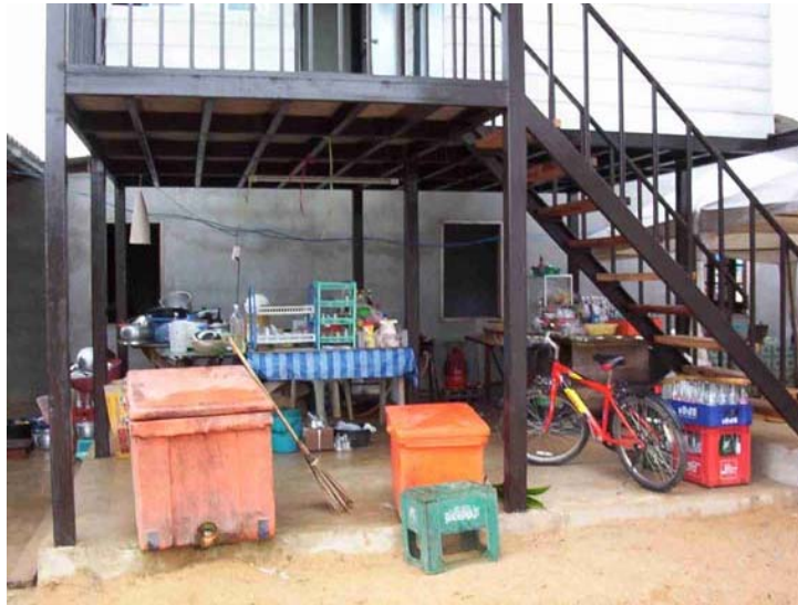
◀ Ground floor of a house which serves as a small food
