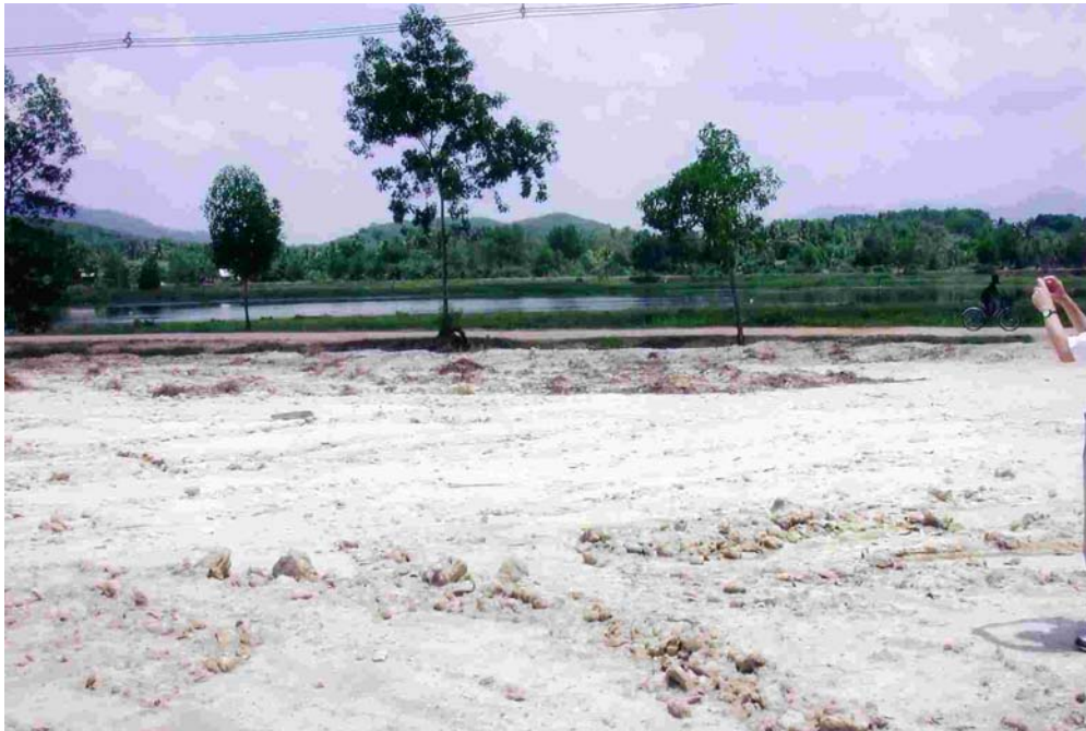
Site of the Construction of 80 Houses in Baan Pru Teow, Phang-Nga
