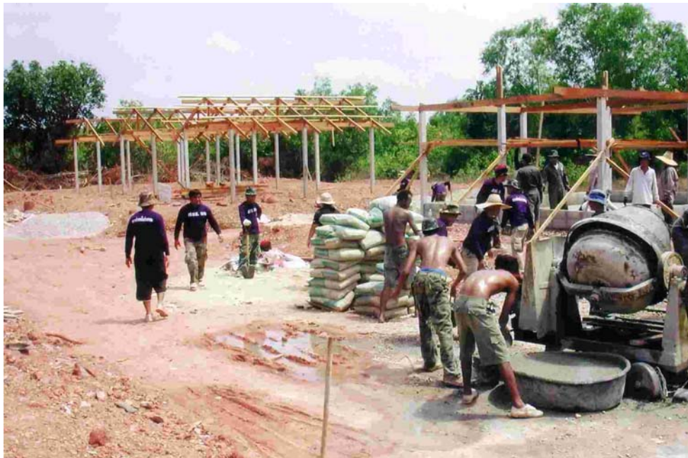
Site of the Construction of 14 Houses in Baan Koh Poo, Krabi
